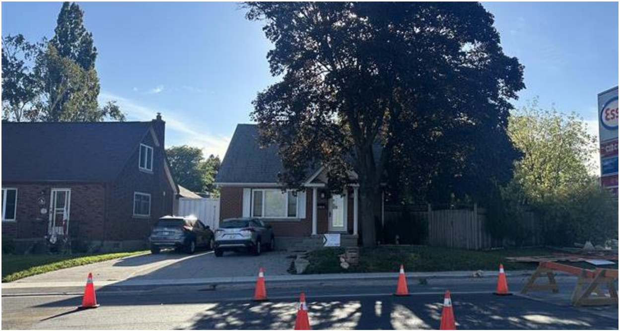
Figure 6: Existing Site Conditions as of October 1, 2025
