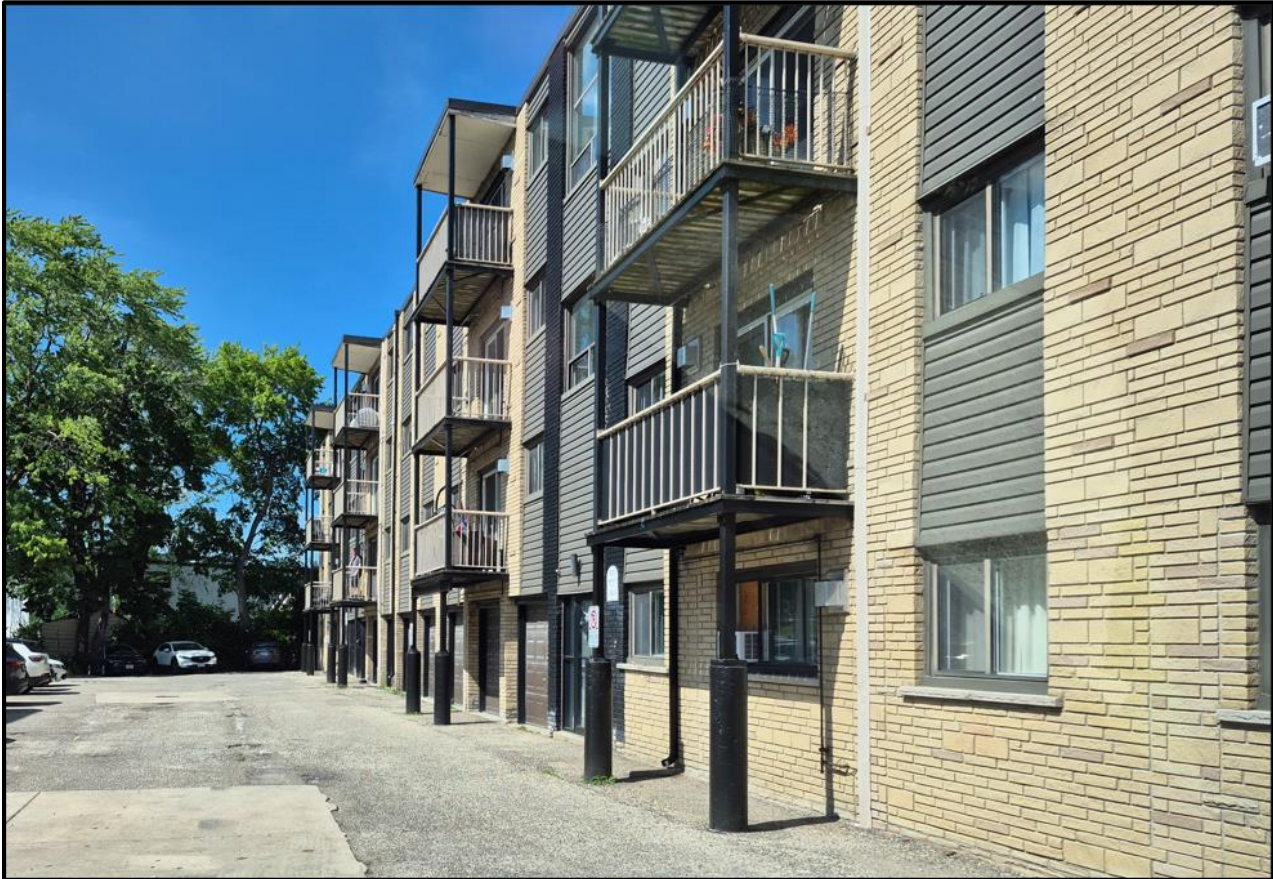
Figure 5: Building # 475, where the Additional Units will be added
