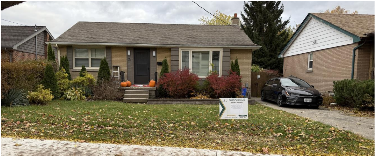
Figure 6: Site photo of 21 Sherwood Avenue.
