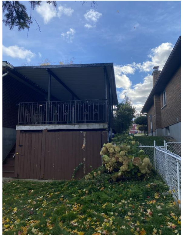
Figure 5: Existing rear deck & roof structure
