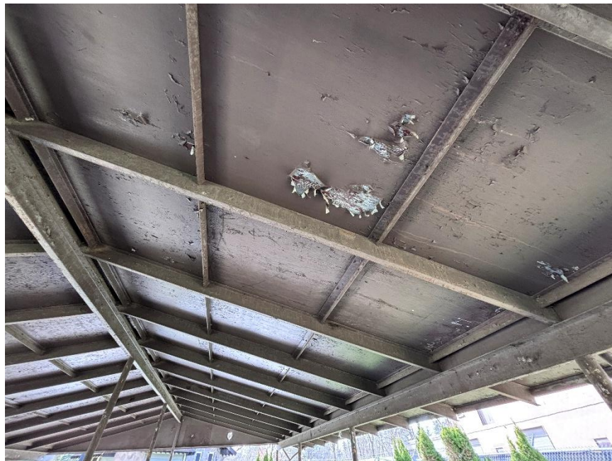
Photo 12 - General view of the roof structure
