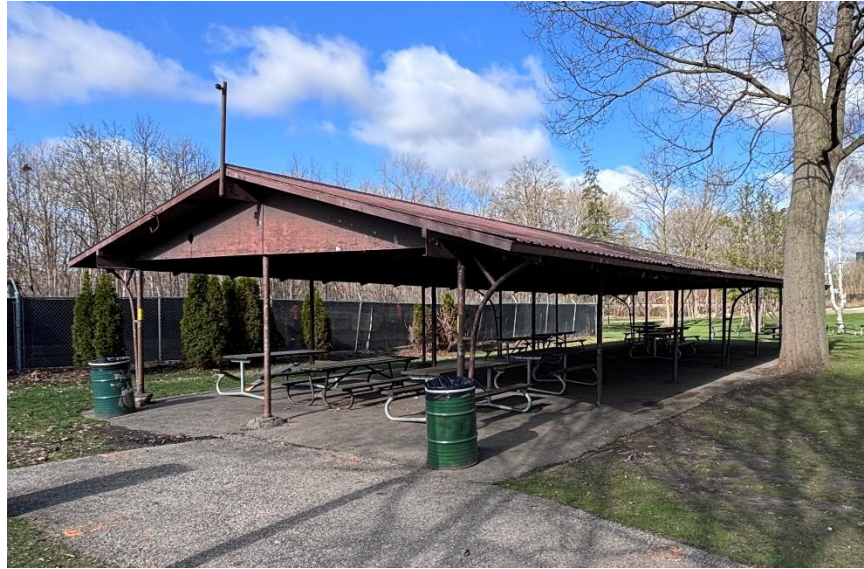
Photo 1 - General view of picnic shelter
