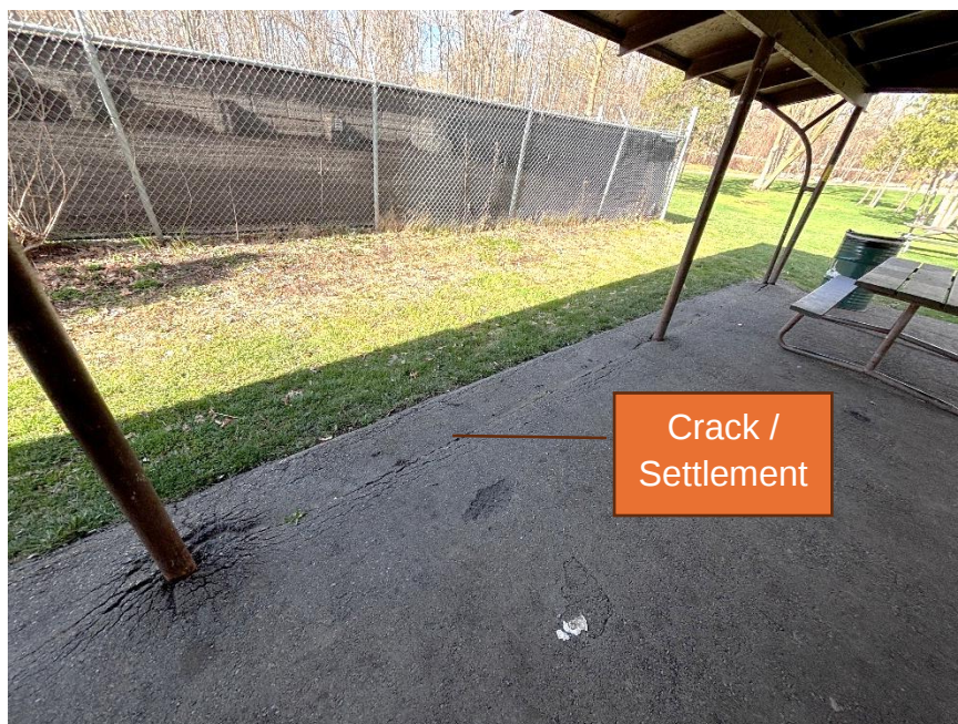
Photo 6 - Deteriorated tarmac
