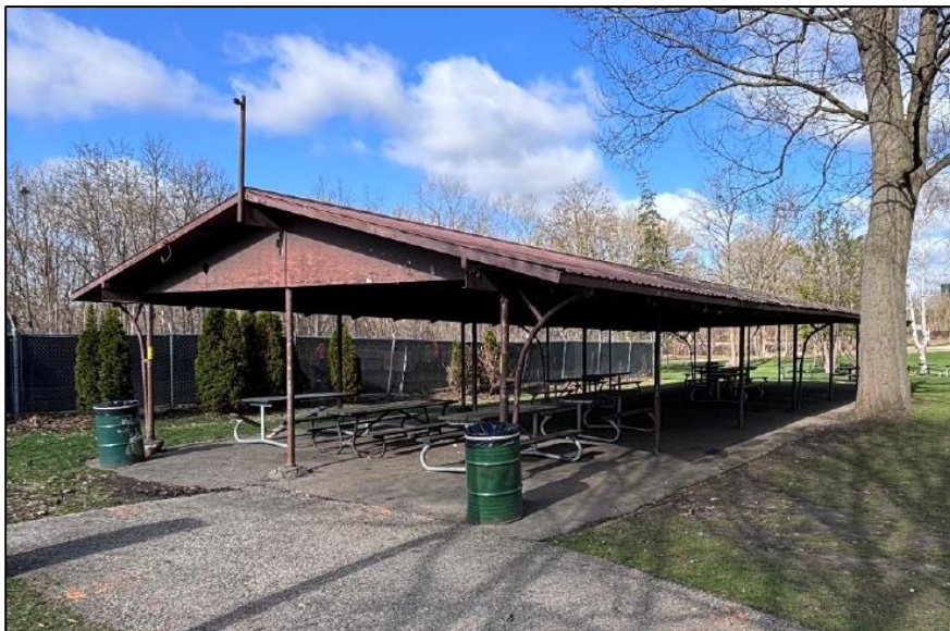
Figure 2: Image of picnic shelter (image source: Structural Condition Assessment report prepared by WitzelDyce Engineering Inc.)
