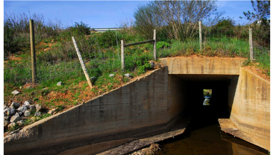
Example of a box culvert for passage of small animals
